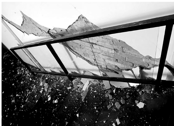
Figure 1. Damaged walls of the Institute of Art History after the earthquake of March 22, 2020. (Photo: Danko Zelić)
